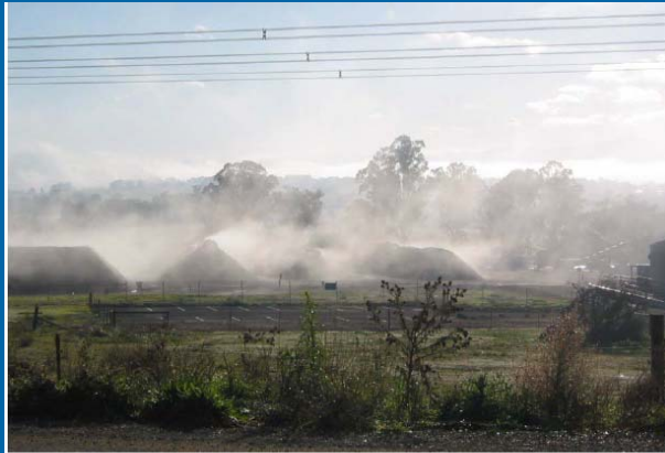
Plate 1. Photograph of water vapour emissions from ANL windrows on the morning of 14 June 2007
